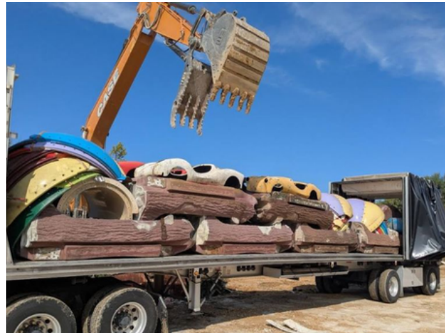
Water slide from a Palace Entertainment waterpark being taken to Veolia's recycling facility.
