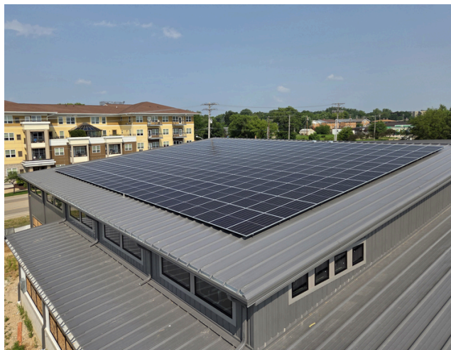
The solar array on the new River Food Pantry building.
