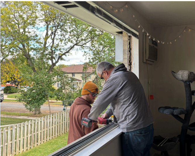
Window replacement at a participating property.
